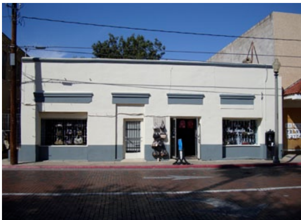
Former José Maria Rodriguez Residence
