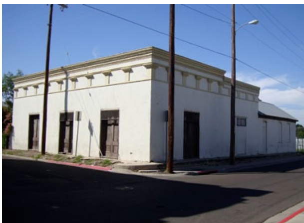
Former Benavides/Herrera Residence
