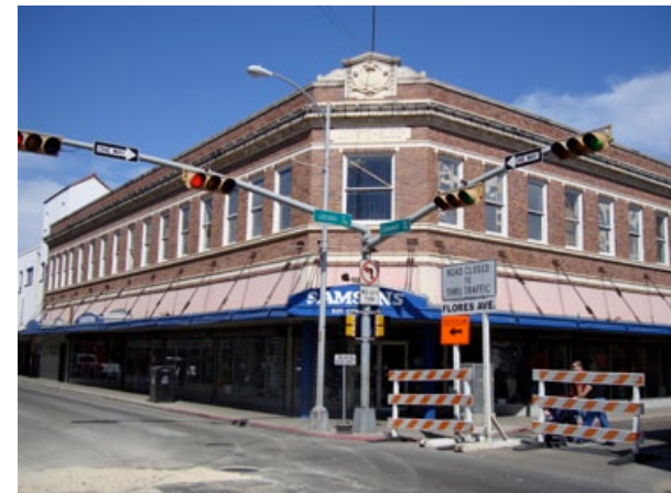
Former Ugarte Building
