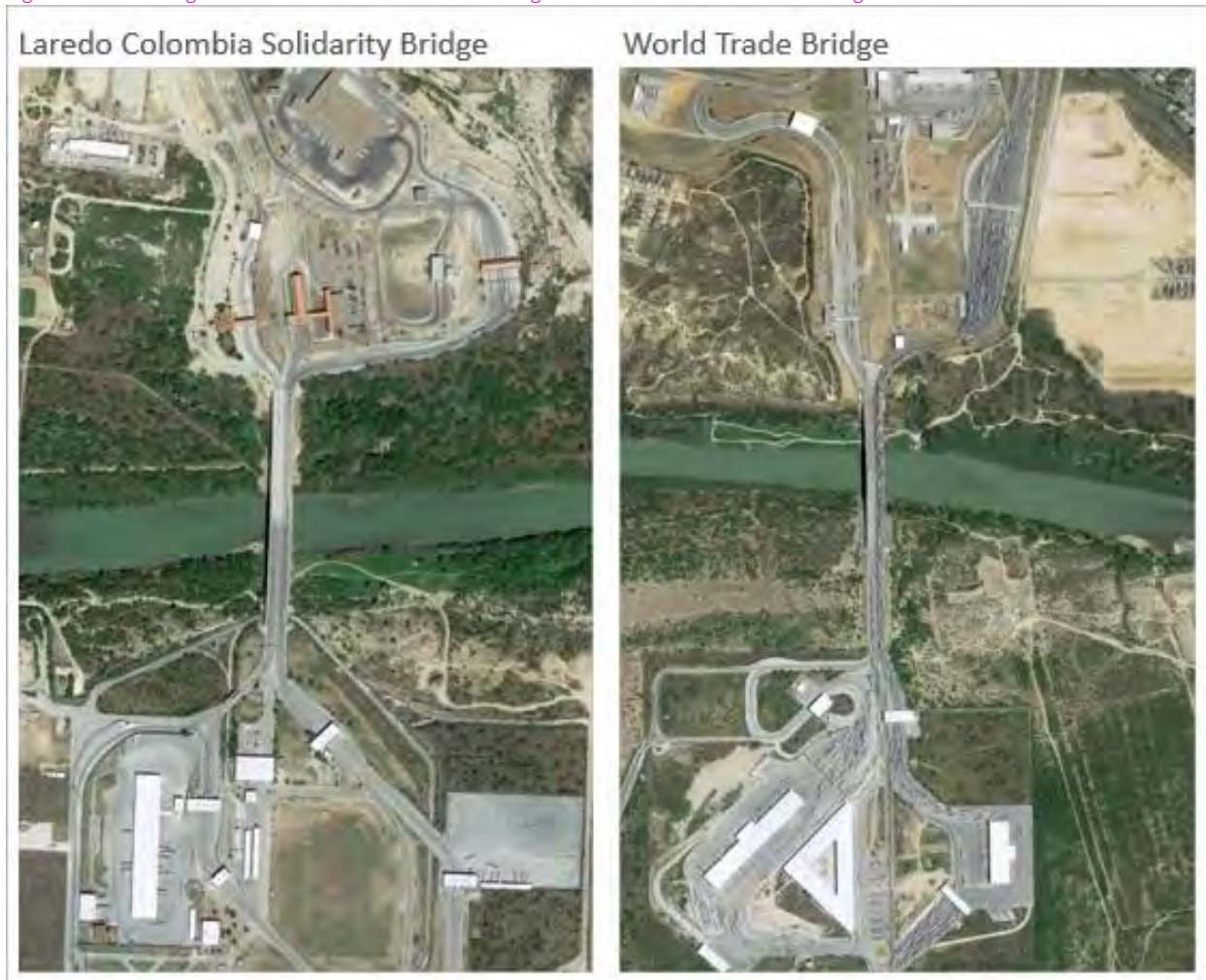
Figure 5. Aerial images of the two commercial truck bridges in the Laredo-Nuevo Laredo region
