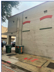
Currently View Condition on Elevation
