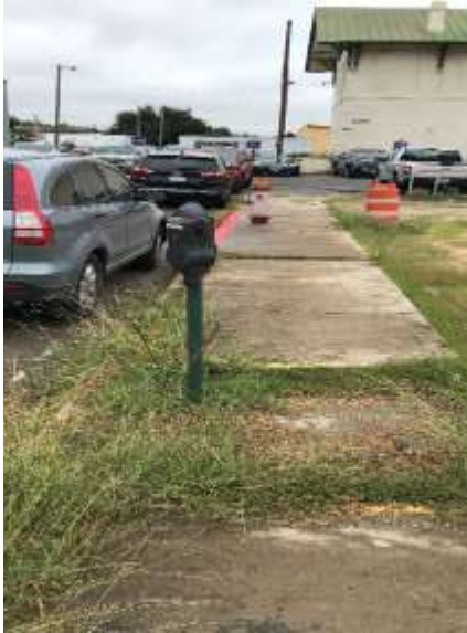
Figure 18: Existing Sidewalk Conditions
