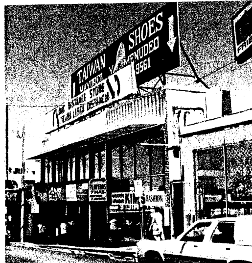
A sign that predominates in the overall building composition is inappropriate.
