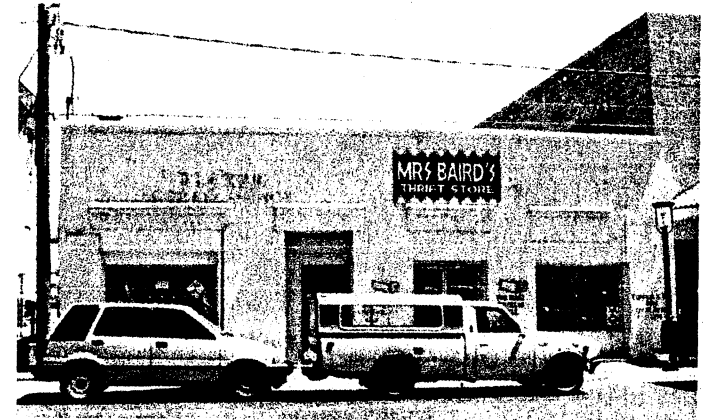
Former José María Rodríguez Residence, 1012 Grant St.
