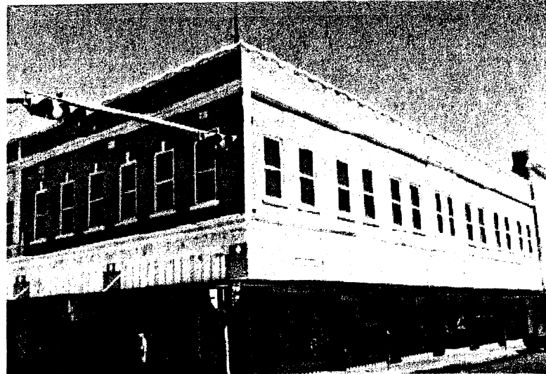
Preserve the character of the roof line.
