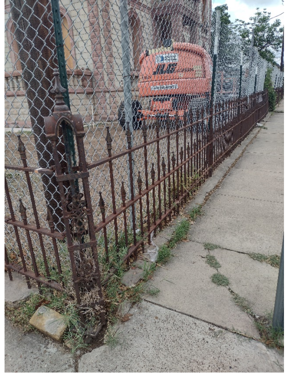
Fence on Davis Avenue
